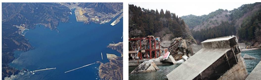
*Figure 11: Damage of the worlds' deepest breakwater in Kamaishi, left before damage, right, after damage* (Source: [www.nytimes.com](http://www.nytimes.com), <http://community.guinnessworldsrecords.com>).
