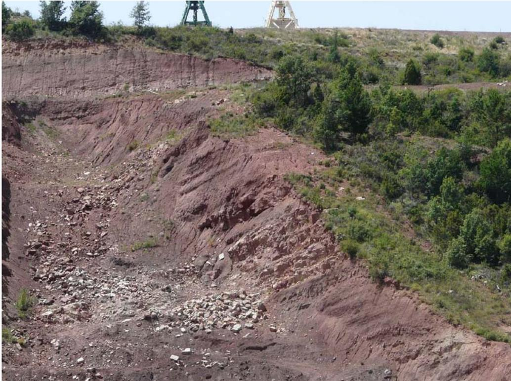
*Figur8-3 - Exposed layer of siltstone and sandstone in the dam abutment excavation.*
