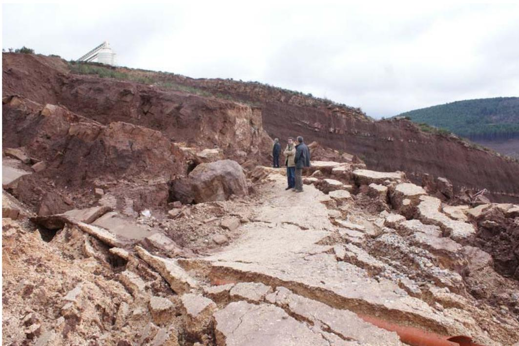
*Figure 8-1 - Failure in the excavated abutments. Downstream, right margin. January 2009.*
