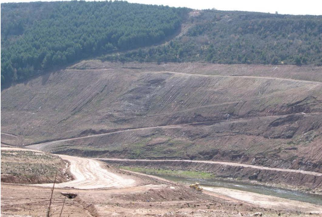
*Figure 8-2 - Shallow landslide in left margin of Arlanza River, upstream of the dam.*
